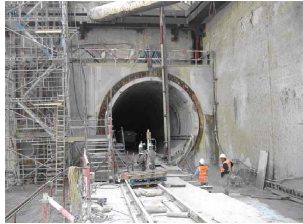
View of the first bore of the tunnel
