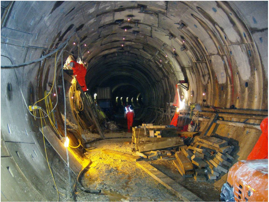
CROSS PASSAGE CONSTRUCTION
